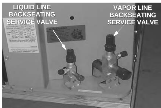
Figure 3 Backseating Service Valves
